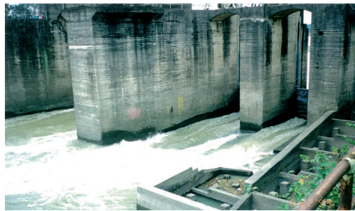
Fig. 5.5.5 Fish ladder at former Rokuzeki Headworks
